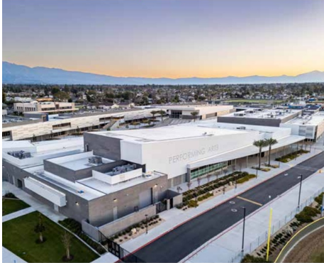
Project: Performing Arts and Gymnasium Buildings, Chino High School, Chino, CA Masonry Contractor: GBC Concrete and Masonry Construction, Inc. Dan Ricketts, MCAC President 2024-2025
