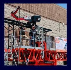
Developed from customer feedback with the needs of the mason in mind, the MULE Rail System is an engineering collaboration between Construction Robotics and EZ Scaffold. This innovation allows a contractor using MULE (Material Unit Lift Enhancer) to quickly and safely move each MULE down a rail system to work another wall section, effectively doubling the amount of wall covered by a single MULE.
